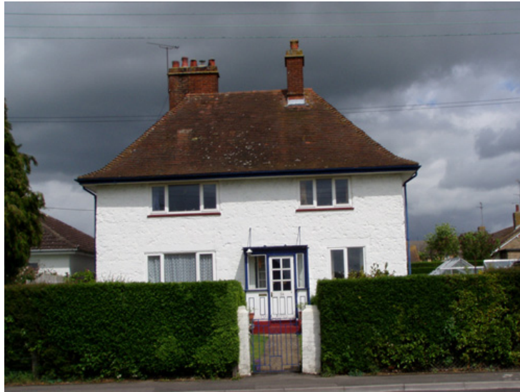
Figure 10.2: Residential rammed chalk property in Amesbury, Wiltshire
