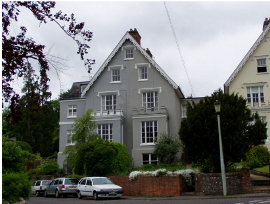
Figure 10.1: Five storey rammed chalk building in Winchester, Hampshire
