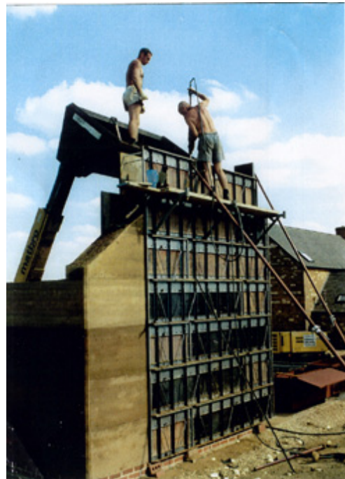
Figure 6.2: Modern Australian Formwork (Bill Swaney)
